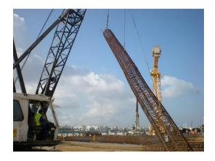
After rotary excavation, the bentonite slurry is recycled and the steel reinforcement cage is lowered down into the pile. The tremie pipe is then installed in the middle of the pile shaft and recycling will continue through the tremie pipe waiting for pouring operations to start.
